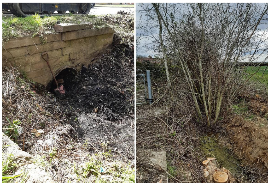
Figure 18: Examples of flow restrictions found through Section 19 investigations (2021)
