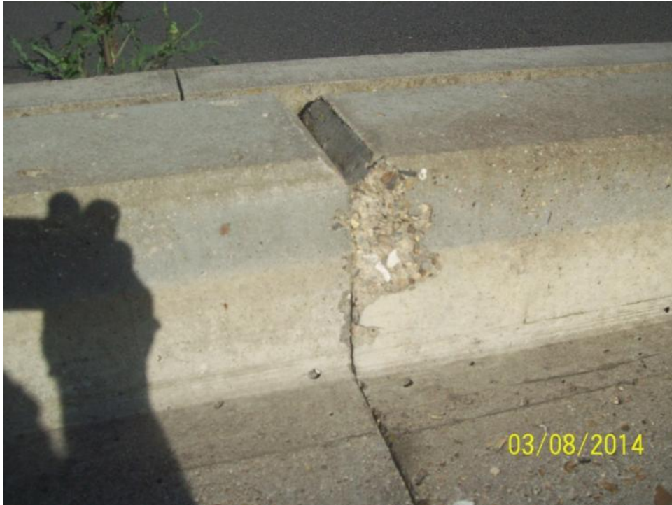
CH41944 S/B – spalling of concrete on upstand (nearside)
