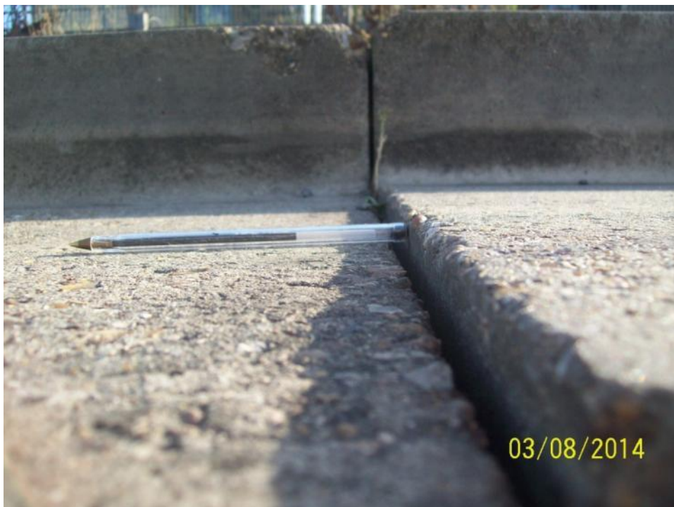
Beam 10 – Dropped beam
