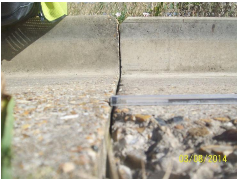
CH60262 H/B – dropped beam (nearside)
