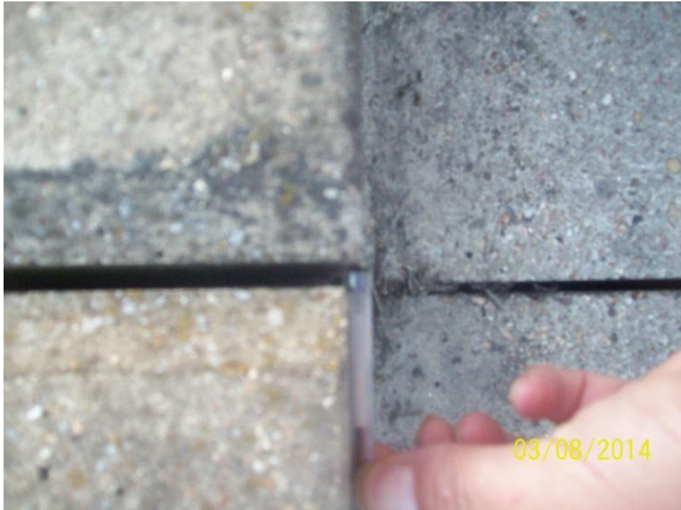
CH17736 C/B – Laterally displaced (nearside)
