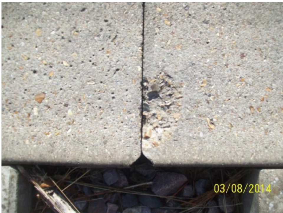
CH41048 P&R/B – spalling of concrete on running beam (nearside)
