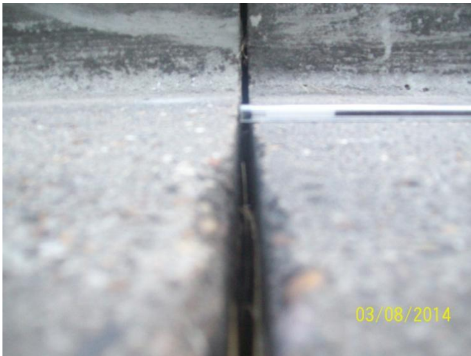
CH17586 C/B – beam dropped
