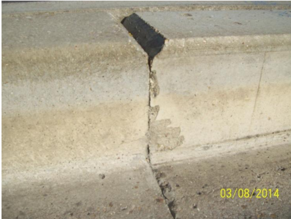
CH42274 S/B – spalling of concrete on upstand (nearside)
