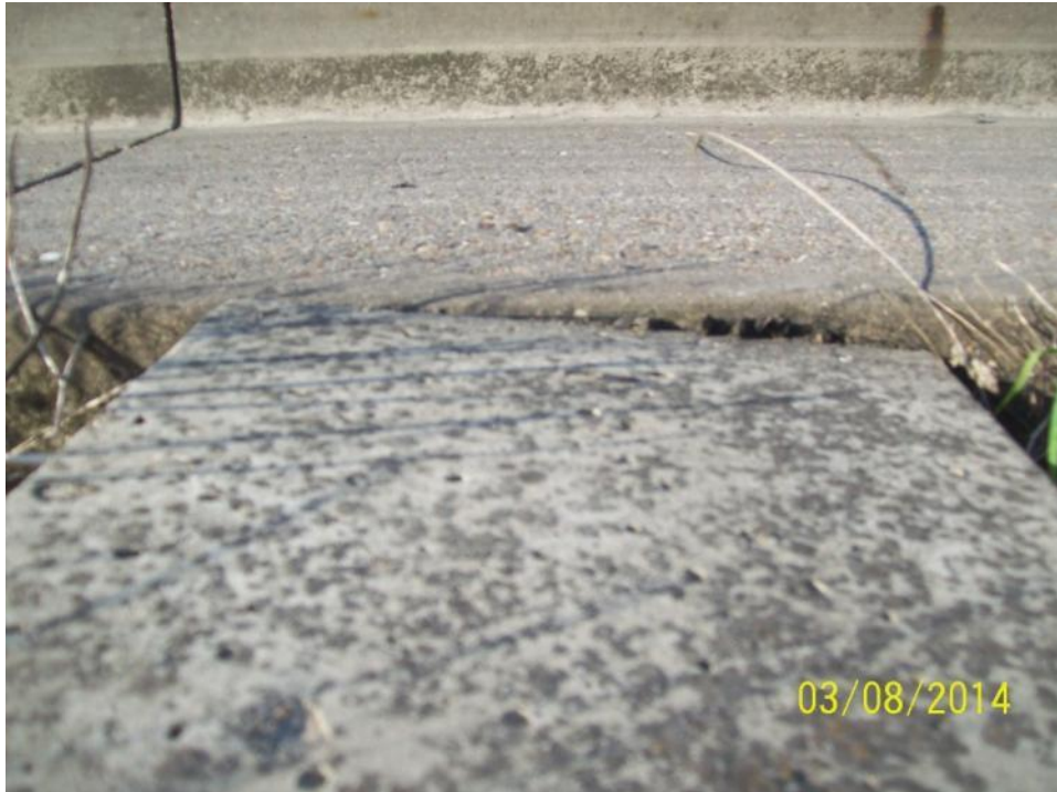
Beam 10 – Twisting spacer beam
