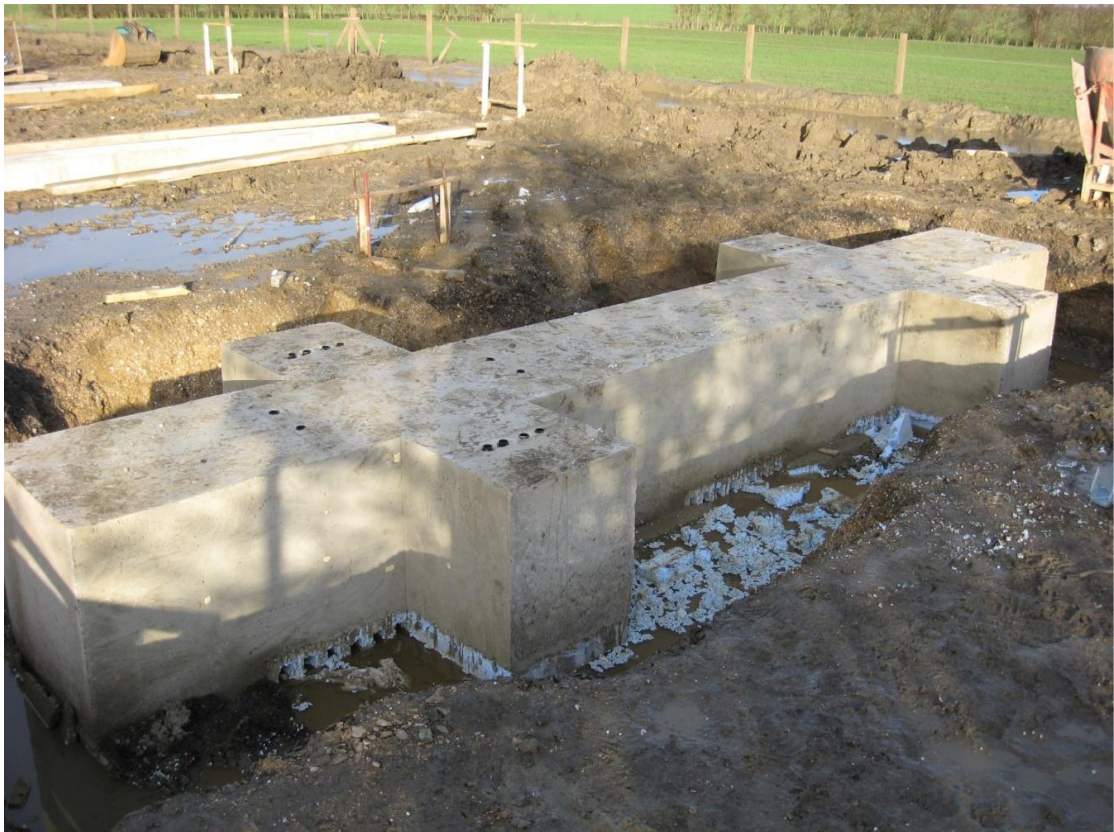
Photograph B2 – Pile Cap Foundation
