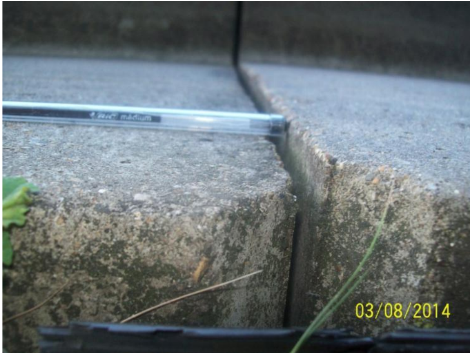
CH18261 S/I B – beam dropped (nearside)
