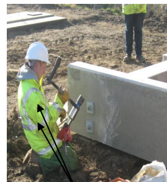
32mm dia connection bolts
