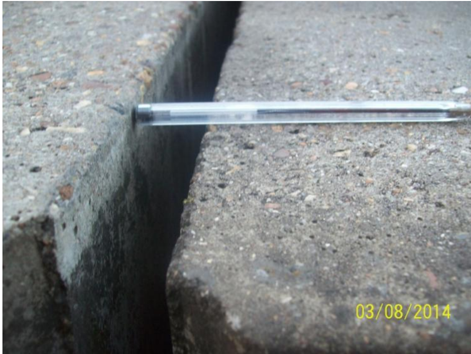
CH17811 C/B – Dropped beam (offside)
