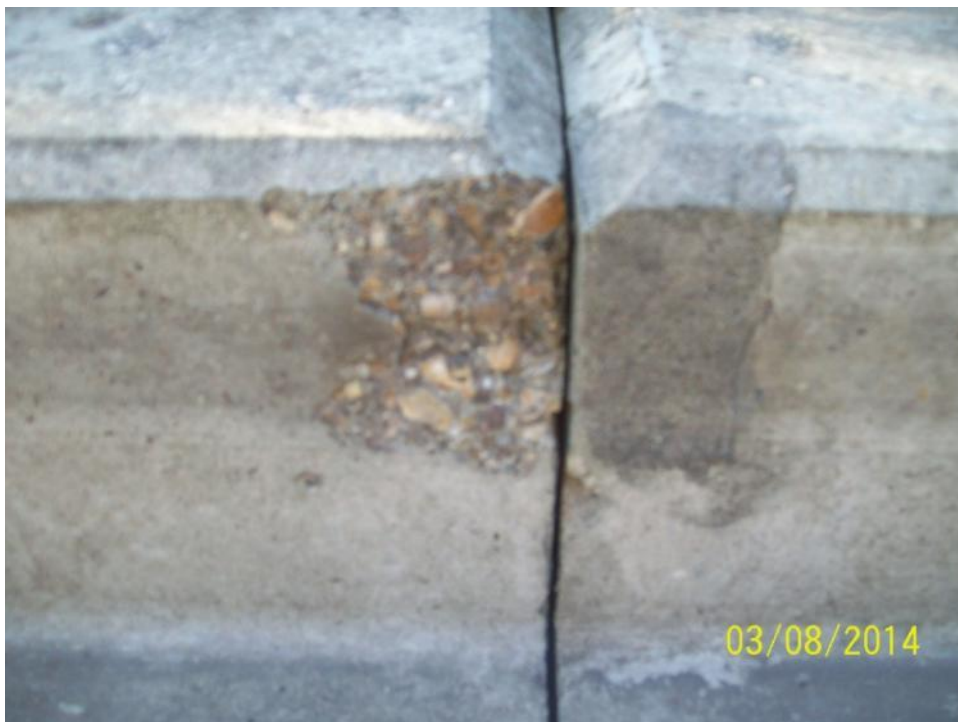
CH43102 – spalling of concrete on upstand
