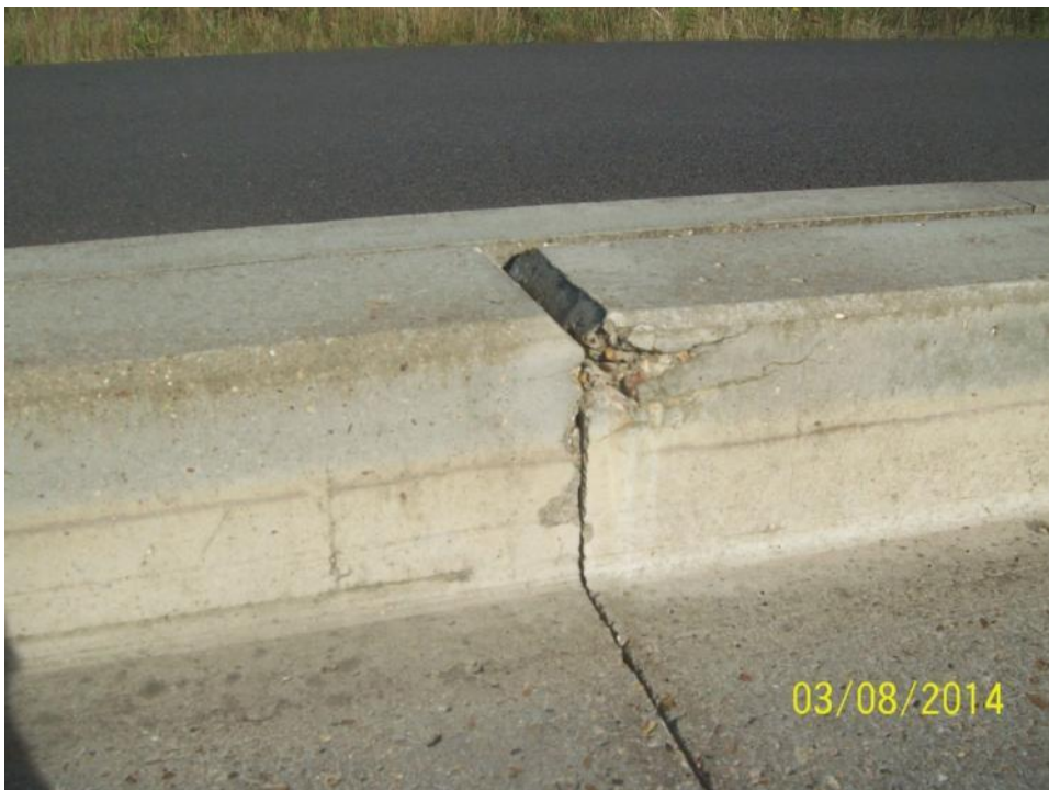
CH42124 S/B – spalling of concrete on upstand (nearside)
