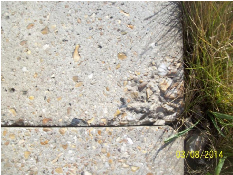
CH60262 H/B - spalling of concrete on running beam (nearside)
