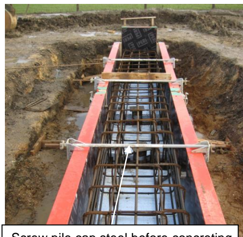
Screw pile cap steel before concreting
