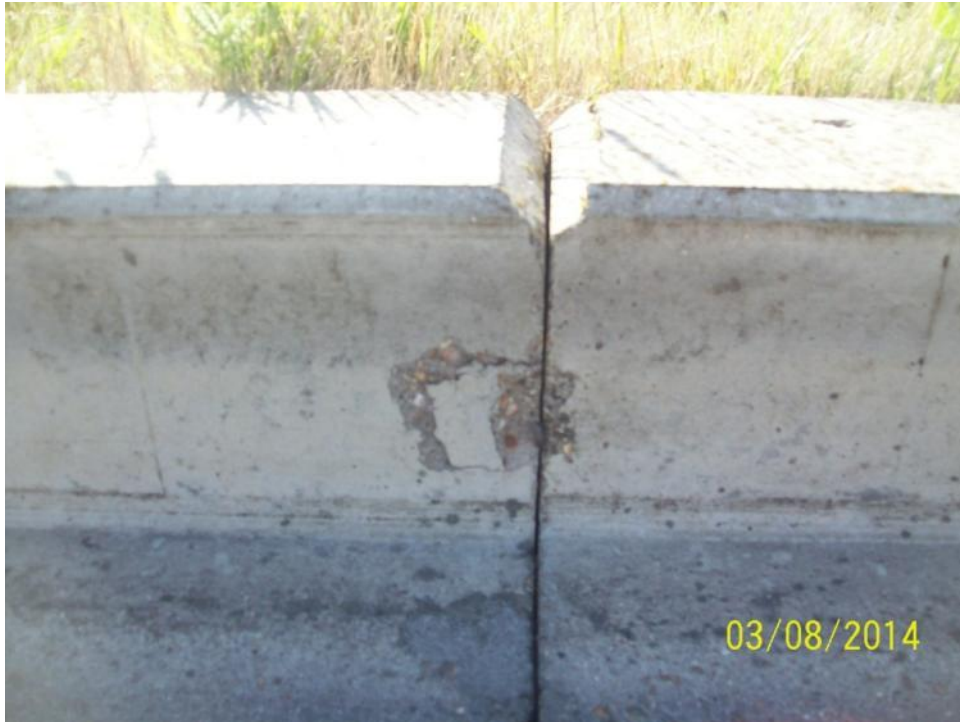
CH42259 P&R/B – spalling of concrete on upstand (nearside)
