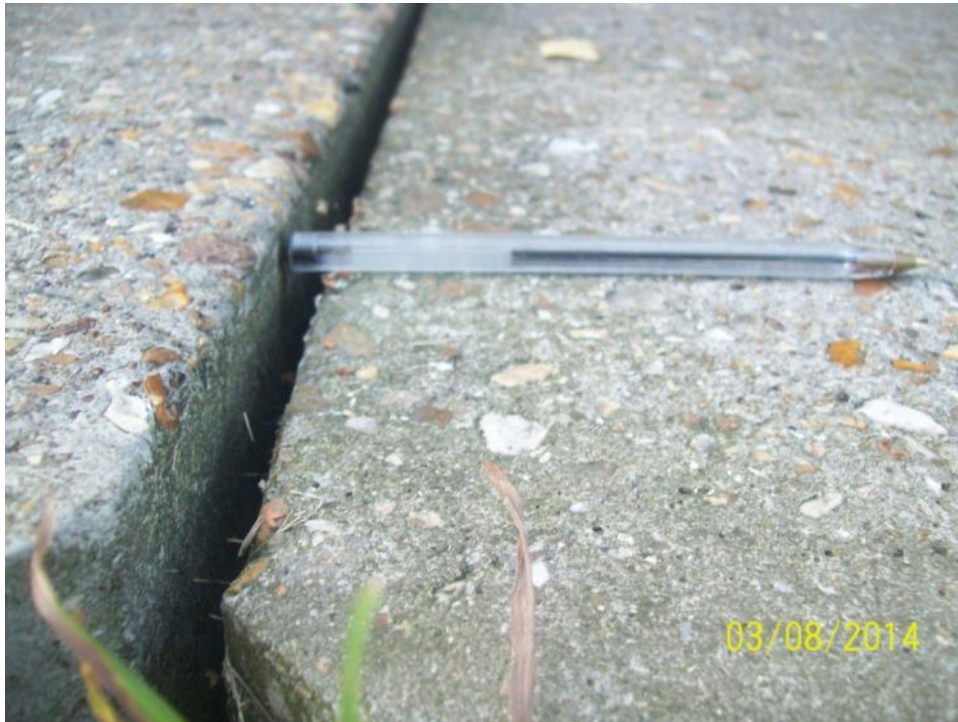
6 th beam from Shelford Rd Bridge towards P&R – dropped beam
