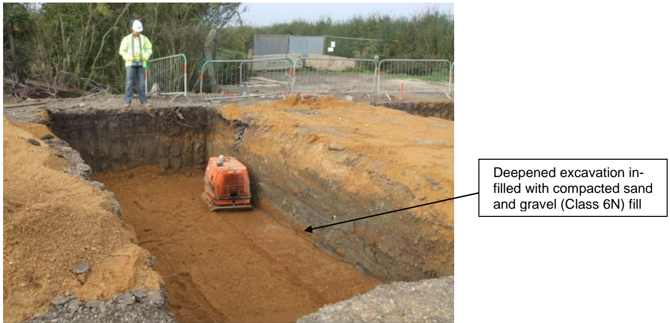
Figure 7. Photograph of an excavation for a shallow foundation that has been filled with Class 6N fill
