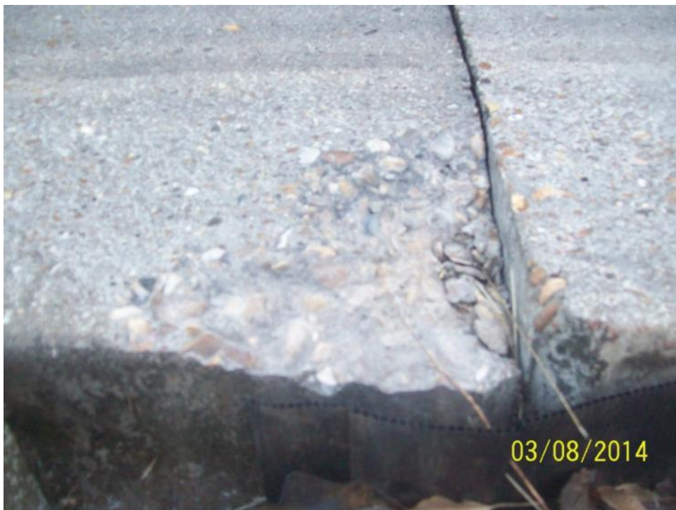
CH17646 C/B – spalling of concrete on running beam (nearside)
