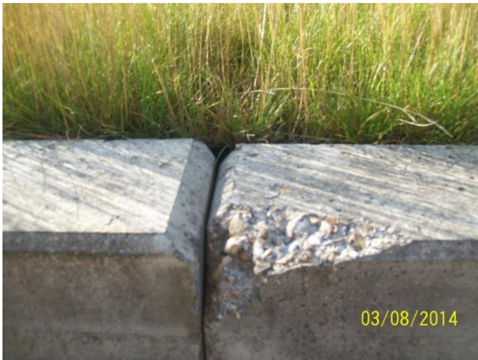
CH43072 - spalling of concrete on upstand
