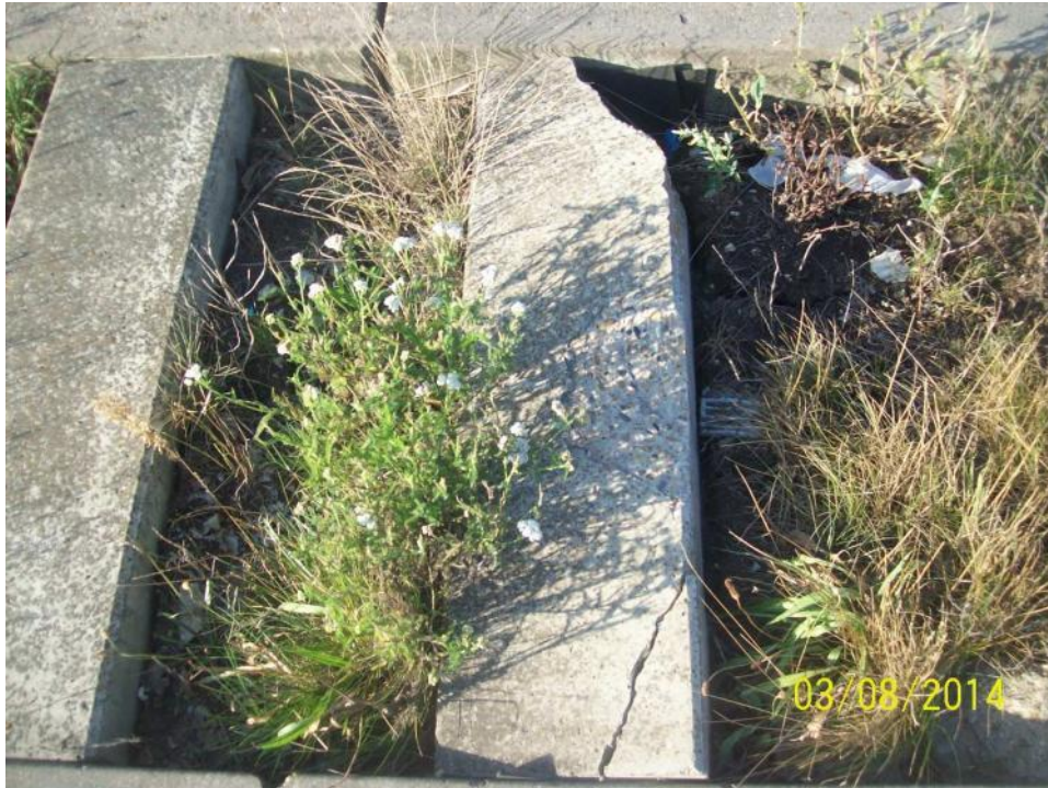
Beam 9 – Broken spacer beam
