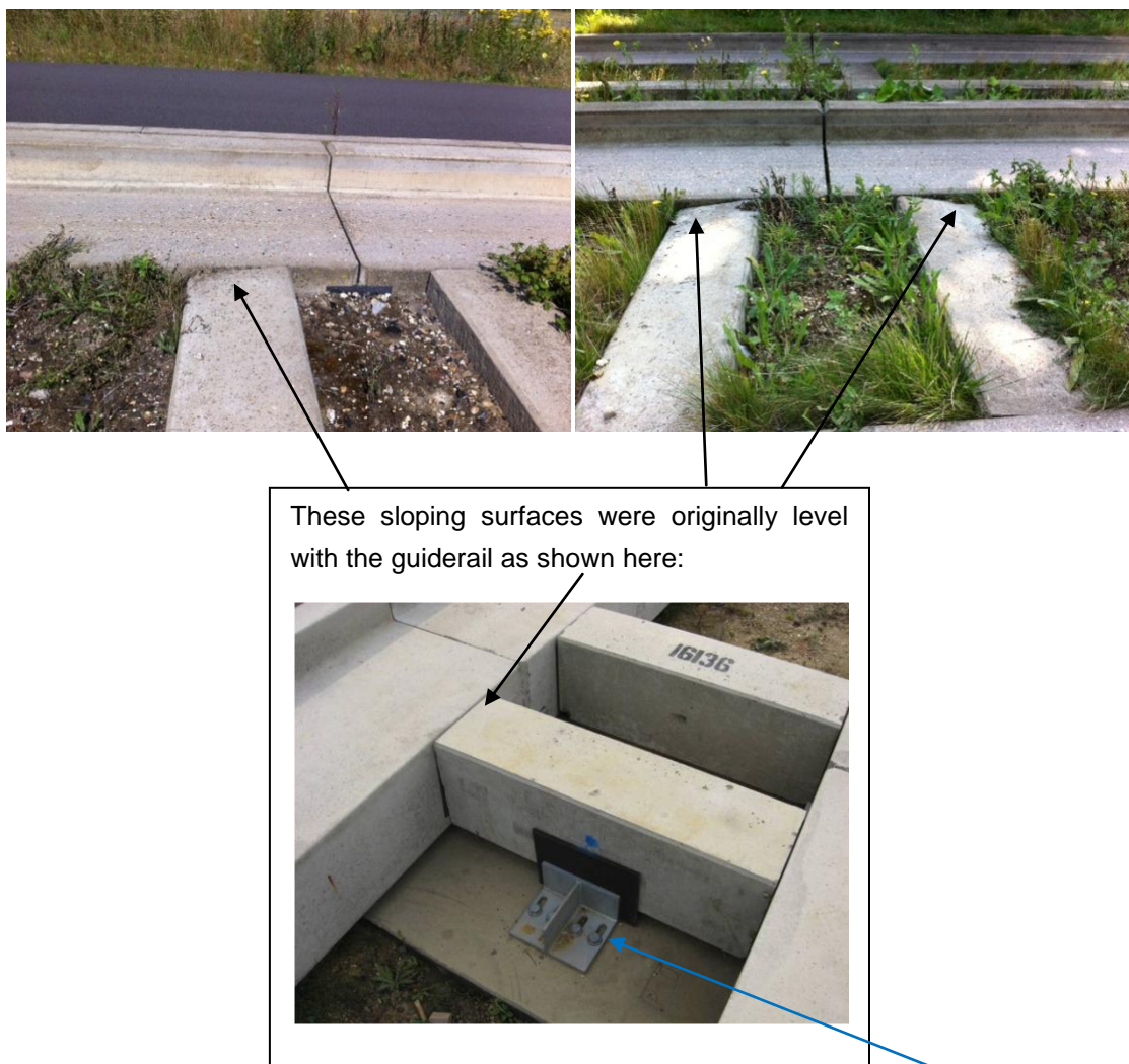
Figure 9. Photographs of rotated spacer beams.
