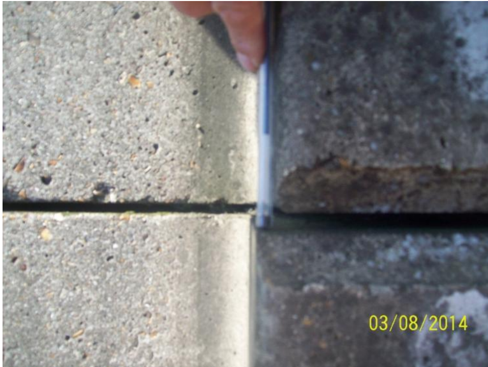
CH17691 S/I B – Laterally displaced (offside)
