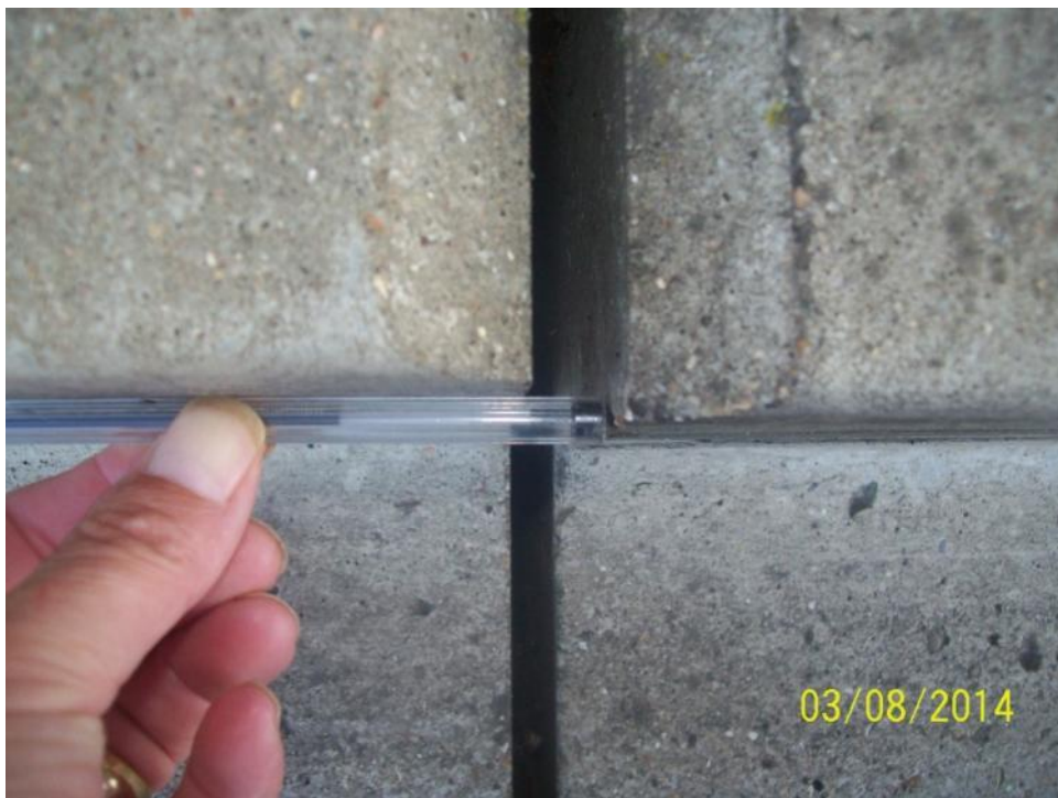
CH17856 C/B – Laterally displaced (offside)
