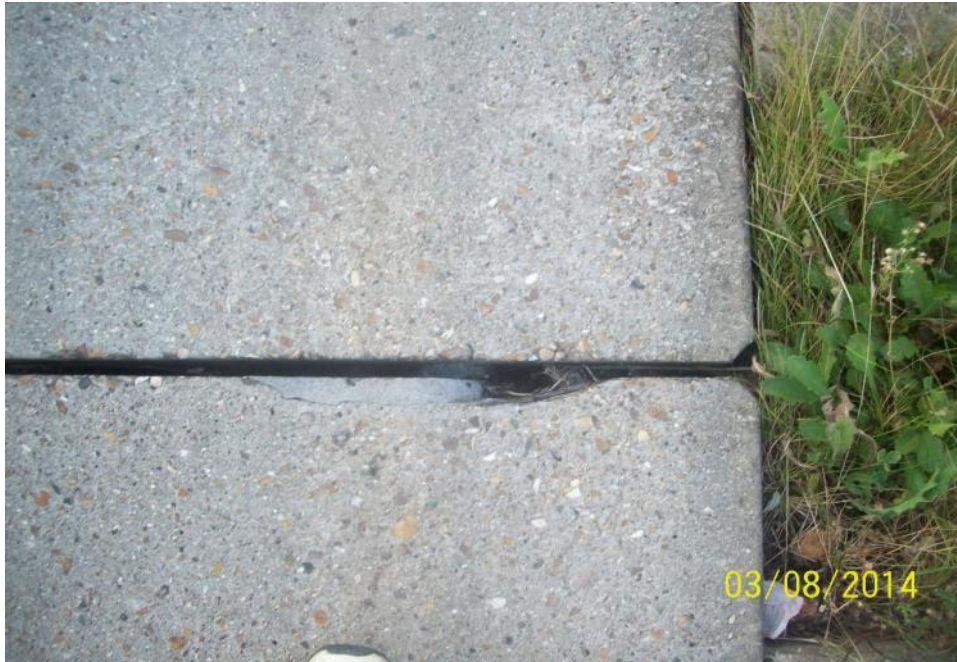
CH19261 C/B – Previous concrete repair has failed (nearside)
