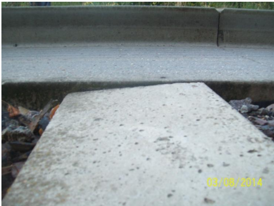
CH17796 C/B – Twisting spacer beam
