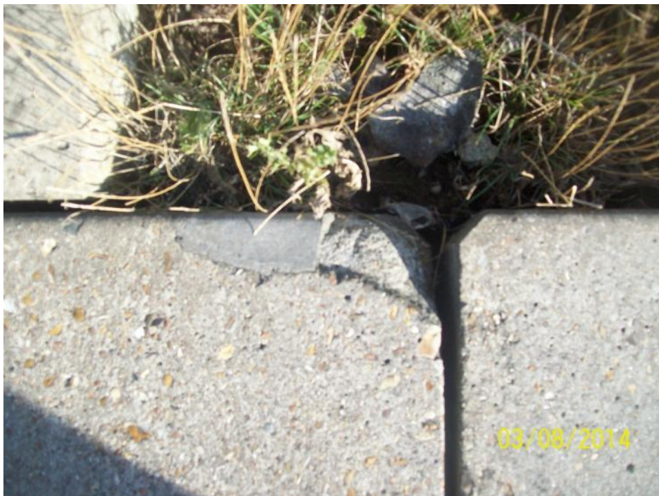
CH42997 – Previous concrete repair has failed
