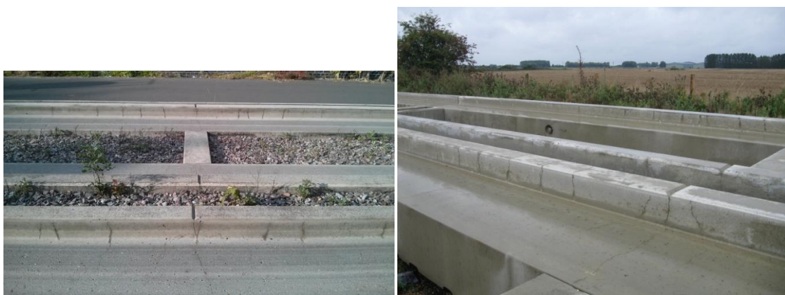
Figure 19. Examples of excessive cracking in guiderrails
