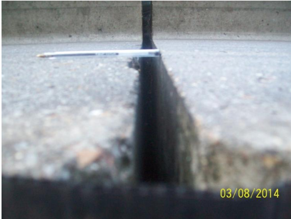
CH17631 C/B – beam dropped (offside)
