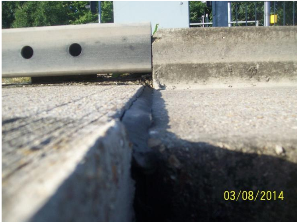
Beam 1 - beam dropped
