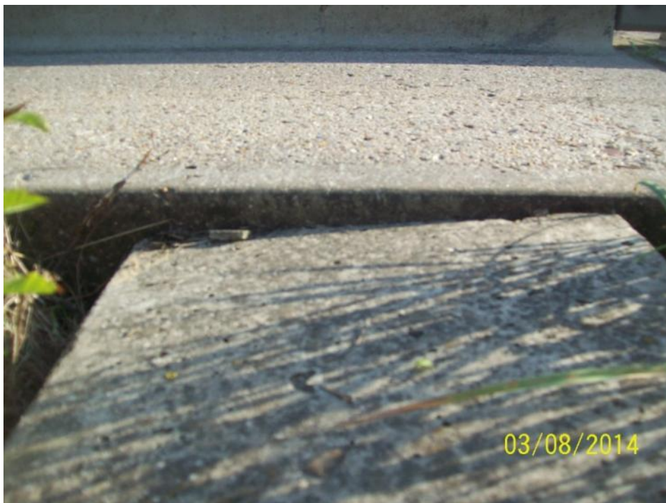
Beam 1 - Twisting spacer beam
