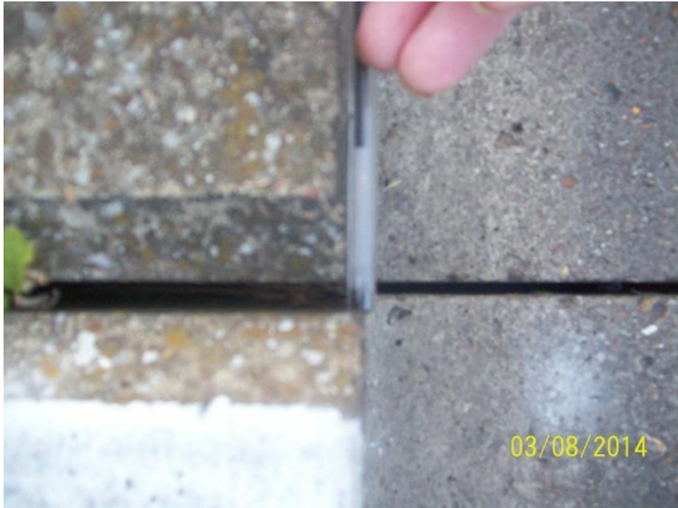
CH17586 C/B – Laterally displaced
