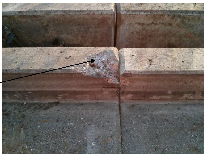
Figure 12. Spalling of concrete.
