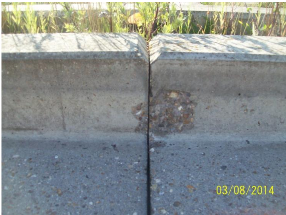
CH42229 S/B – spalling of concrete on upstand (offside)
