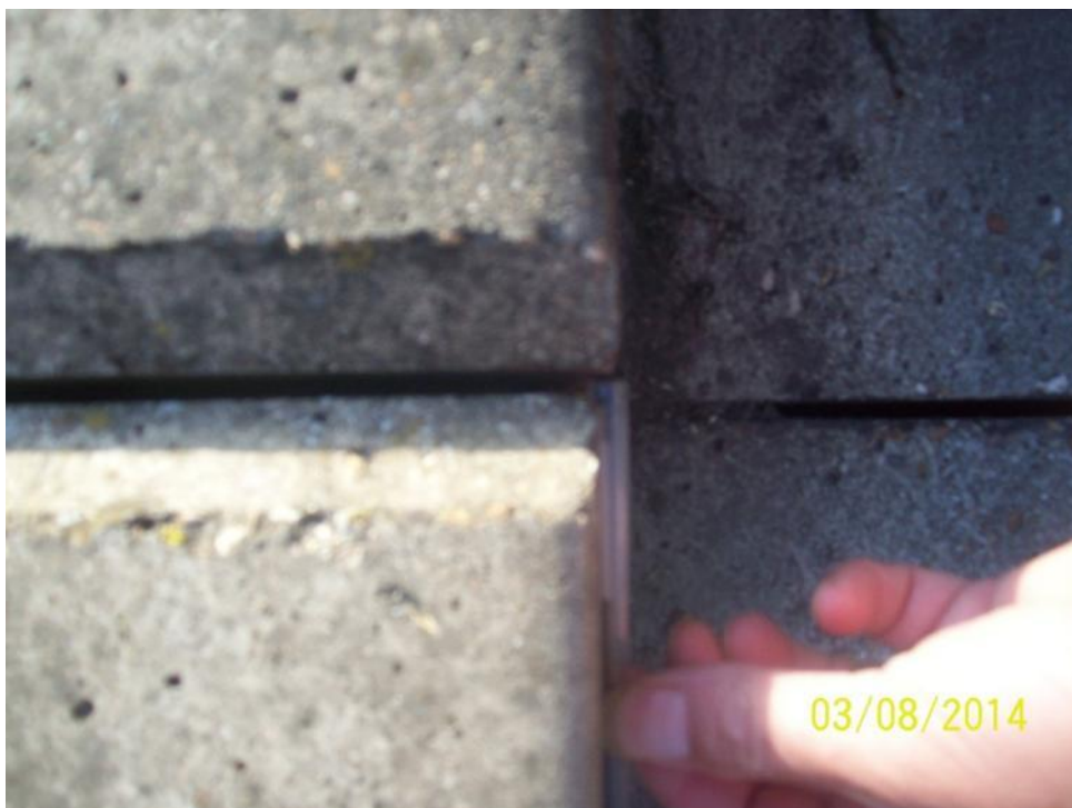
CH17706 C/B – Laterally displaced (nearside)
