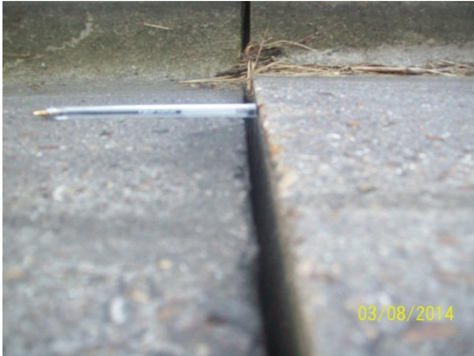
CH17586 SI/B – beam dropped (nearside)
