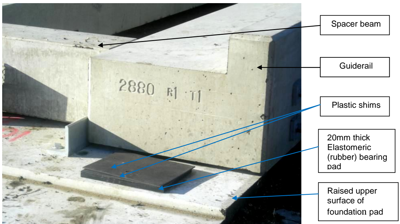
Figure 2. Photograph of a part of the guideway during construction, showing a spacer beam, guiderail, shims, bearing pad, and foundation pad.
