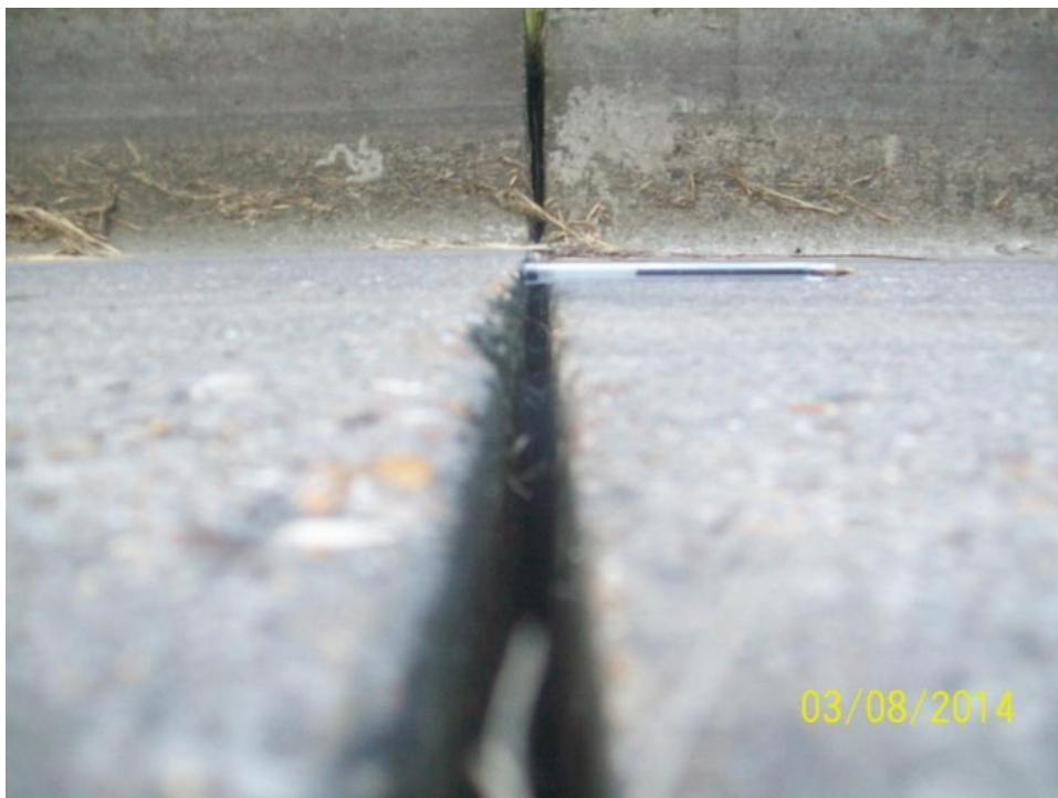
CH17631 SI/B – beam dropped (nearside)
