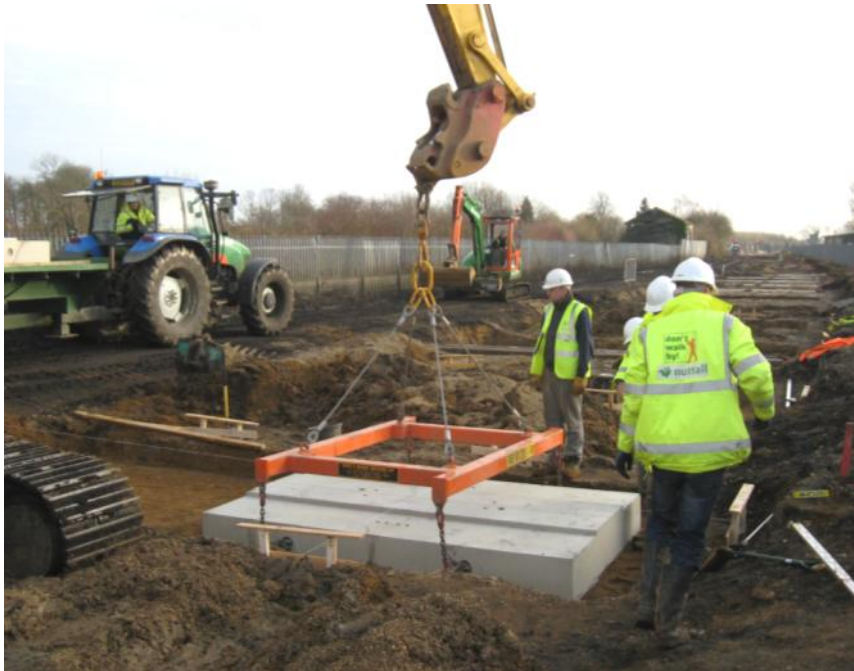
Figure 8. Photograph of a foundation pad being placed.
