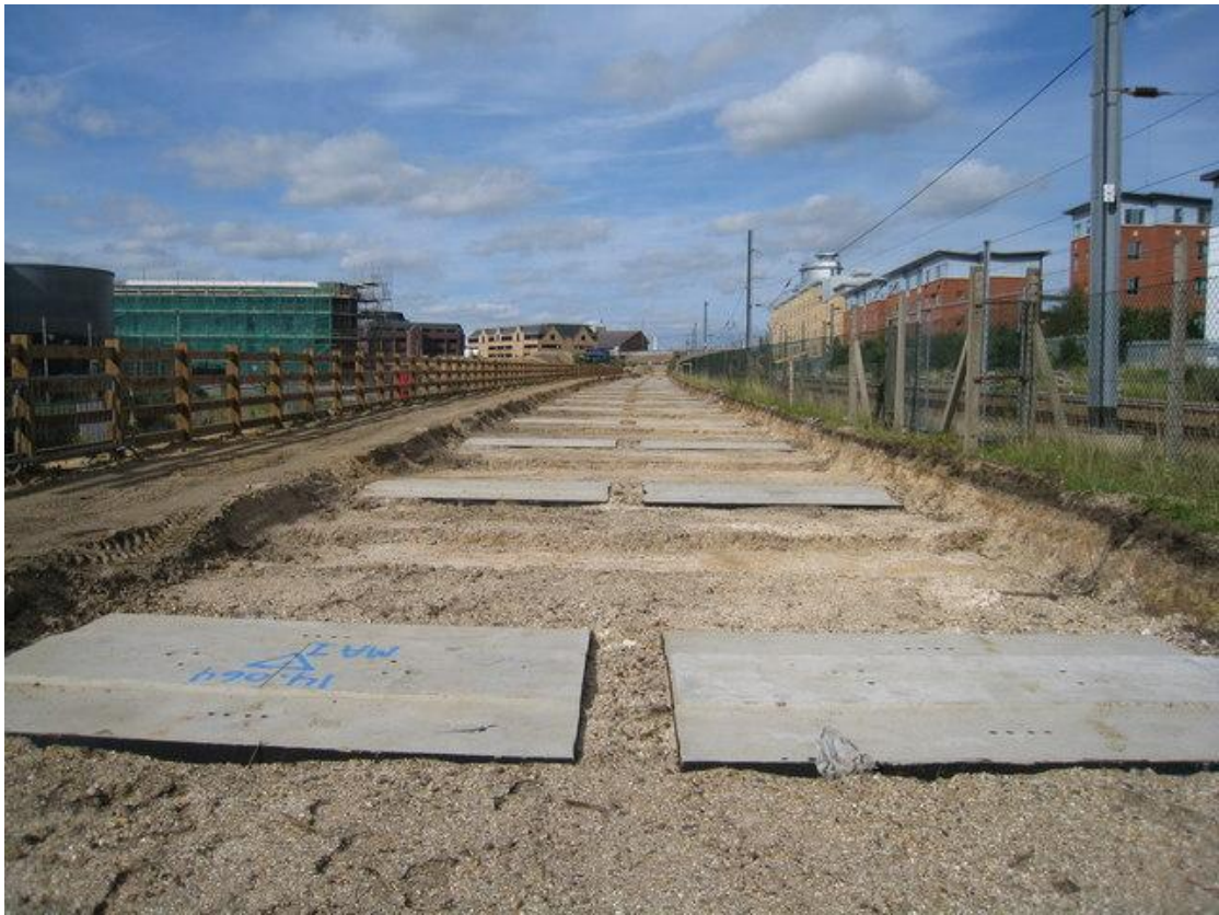
Photograph B1 – Foundation pads
