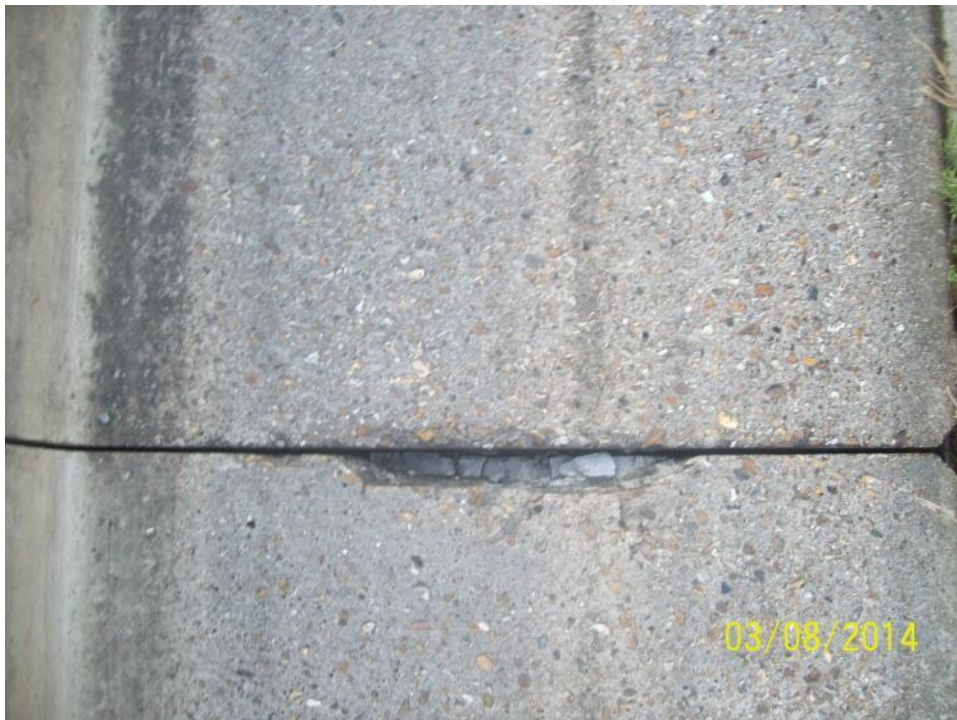
CH18876 C/B – Previous concrete repair has failed (nearside)
