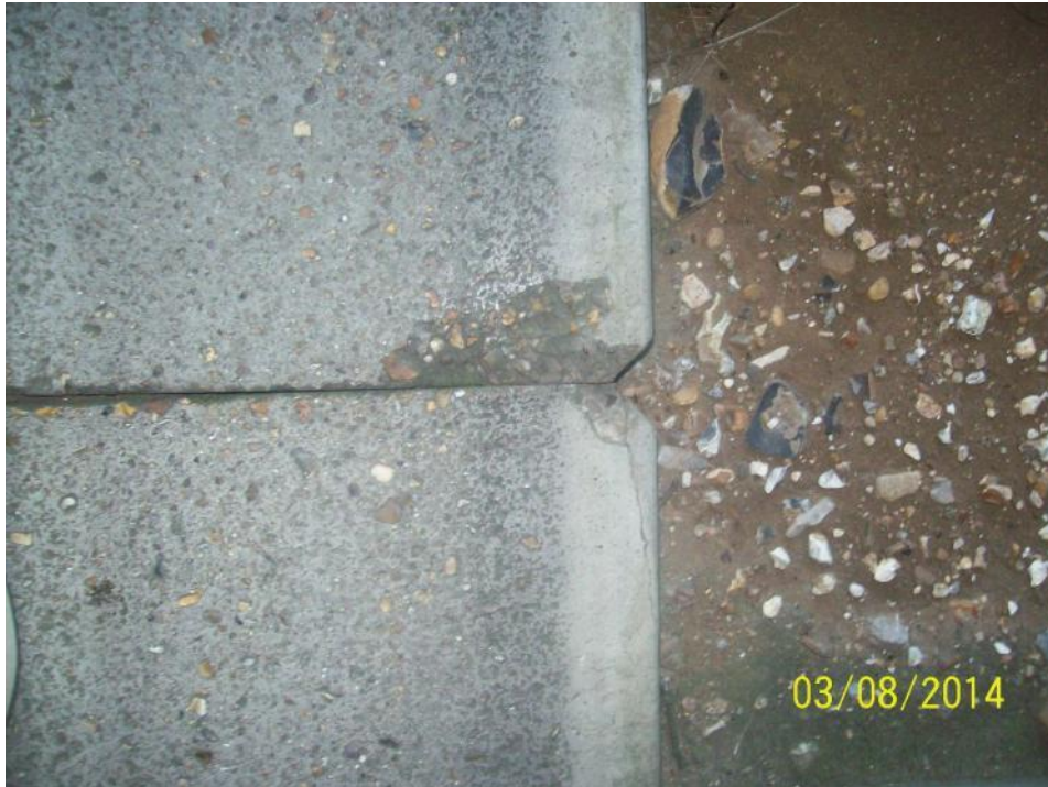
CH18786 C/B – Spalling of concrete on running surface (offside)
