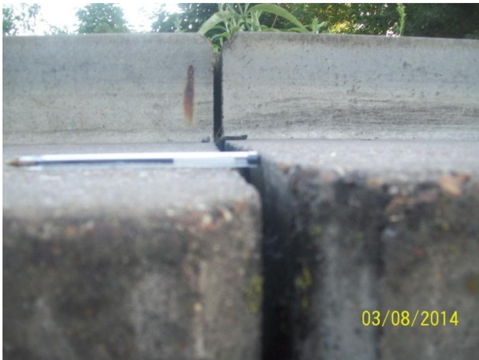
CH17751 C/B –beam dropped (nearside)
