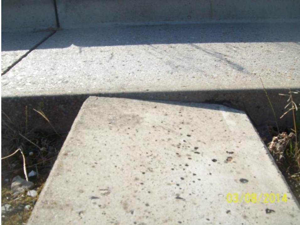
CH42199 S/B – Twisting spacer beam
