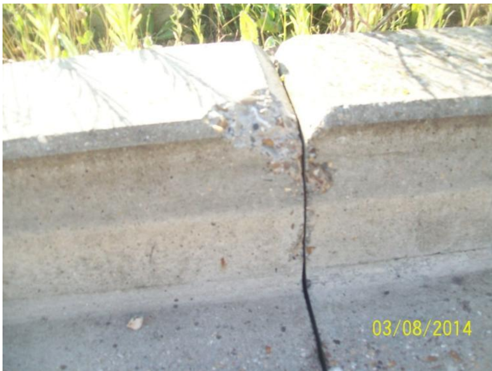
CH42259 S/B – spalling of concrete on upstand (offside)
