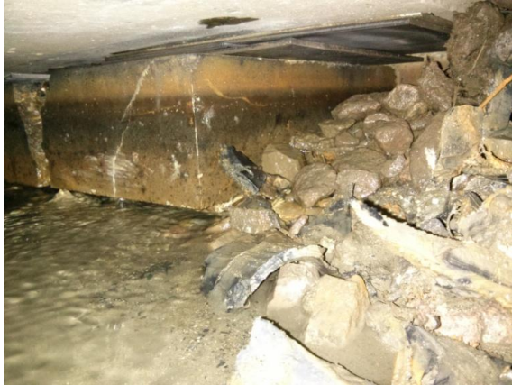
Figure 14. Photograph showing cracked block and displaced shims
