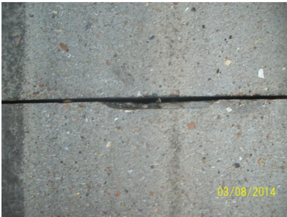
CH18756 C/B – Previous concrete repair has failed (nearside)
