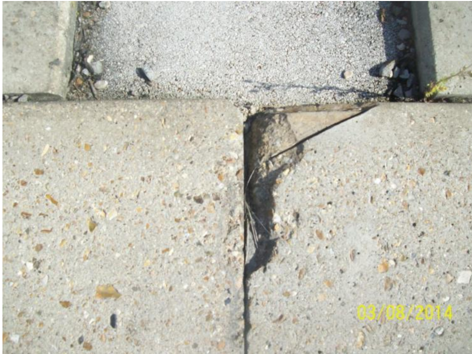
CH60387 H/B – spalling of concrete on running beam (offside)
