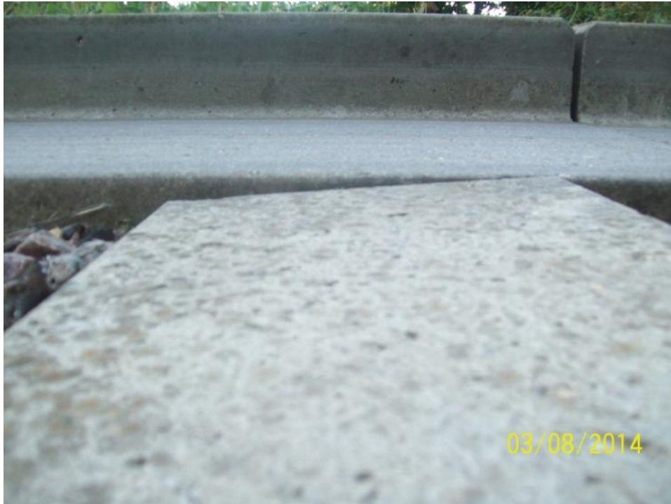
CH177796 SI/B – Twisting spacer beam
