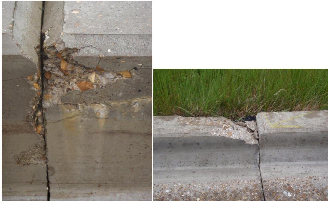
Figure 18. Two examples of spalling.
