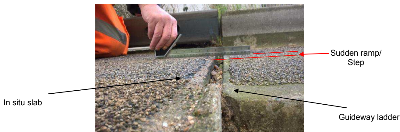
Figure 22. Step at joint between guiderail and insitu slab
