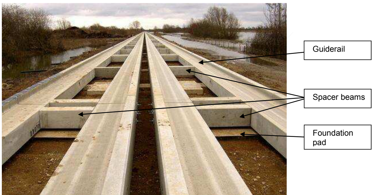
Figure 1. Photograph of a section of the guideway showing the spacer beams and foundation pads.
