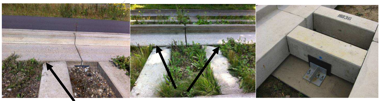
Figure 18. Photographs of rotated spacer beams. The marked sloping surfaces in the two photographs to the left were originally level with the guiderail as shown in the far right photograph.
