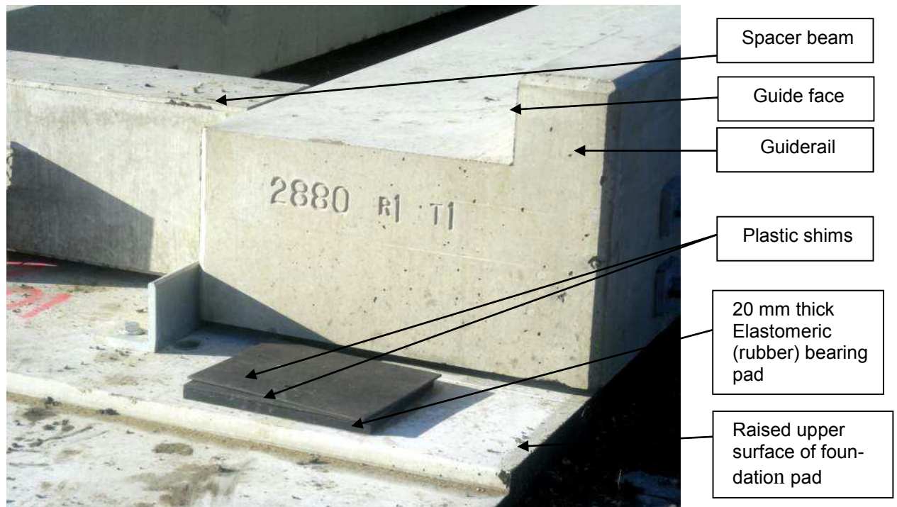
Figure 2. Photograph of a part of the guideway during construction, showing a spacer beam, guiderail, shims, bearing pad, and foundation pad.
