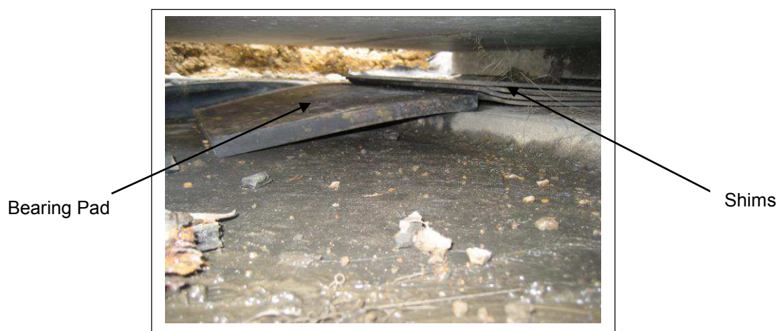
Figure 11. Bearing pad has 'walked out' from beneath the shims.
