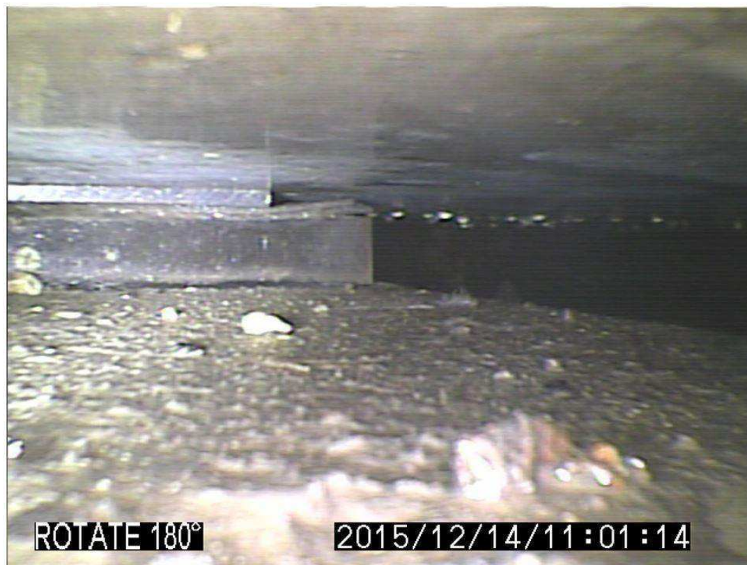
Figure 16. Uneven compression of Elastomeric Bearing Pad.
