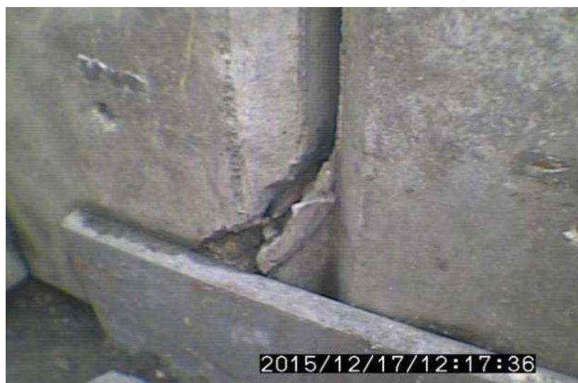
Figure 20. Spalling behind lateral restraint bracket
