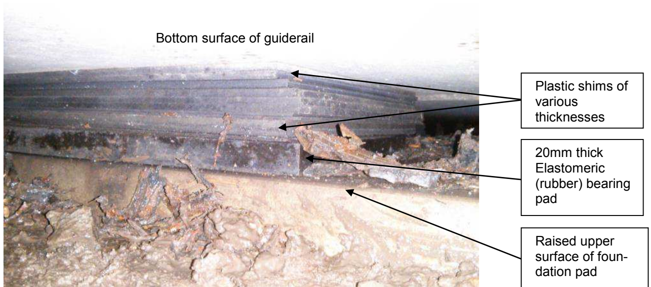
Figure 3. Photograph of a foundation pad upon which there are more than 35mm of shims.
