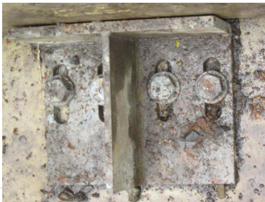
Figure 19. Photograph showing longitudinal bracket not abutting spacer beam.
