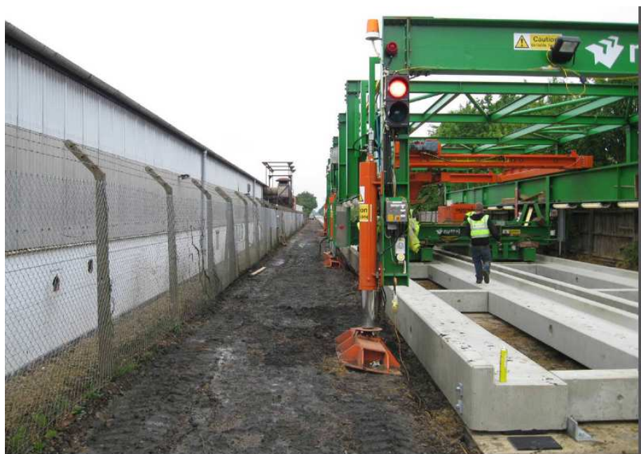
Figure 2 – Gantry Laying PCC Units
