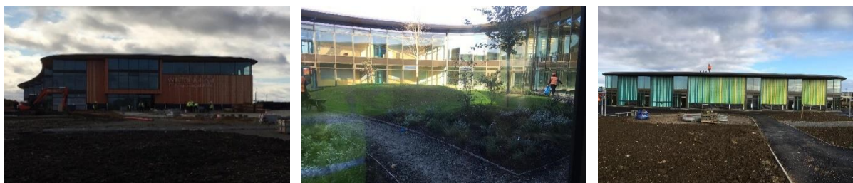
New Build: Wintringham Primary Academy
