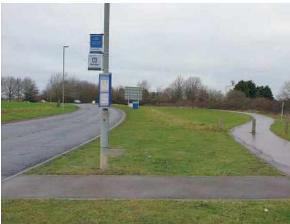
Photo 39: Section of footway across verge to access bus provided retrospectively several years after bus stop became operational, Cambourne.
