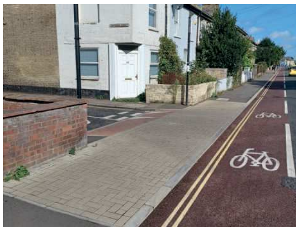
Photo 13: Continuous footway for pedestrians, Histon.
