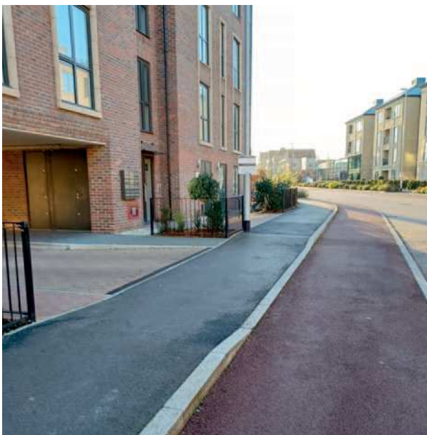
Photo 16: Continuous footway and cycleway across car park access, Darwin Green, Cambridge.
