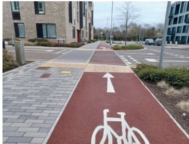
Photo 22: Side road crossing which keeps kerb lines giving the feel of a traditional junction contrary to the give way markings. Design should reinforce the priority, Eddington, Cambridge.
