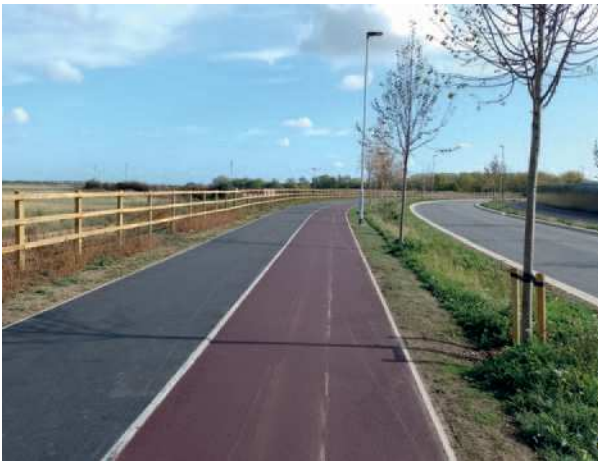
Photo 5: Segregated cycleway and footway on each side of the carriageway on a primary street, Waterbeach New Town. Dedicated space considered for pedestrians and cyclists, and lighting along the route.
