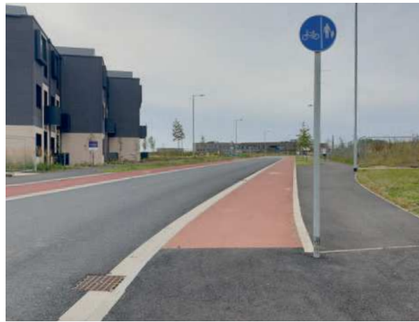
Photo 20: Stepped cycle lane on each side of the carriageway on a primary street, Northstowe Phase 2 (it is recommended to put signs on wooden bollards (see photo 49) or existing posts to reduce street clutter).
