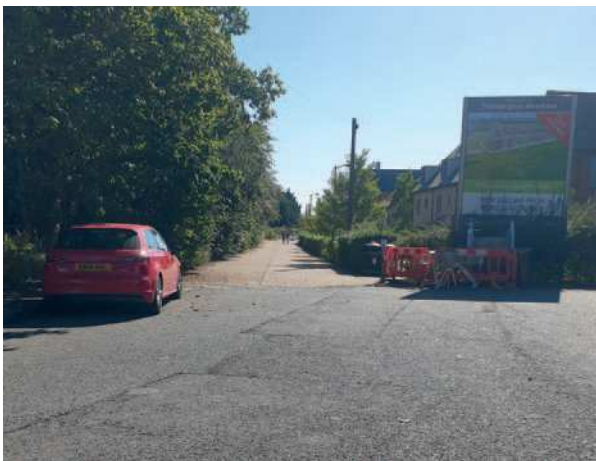
Photo 11: Poor provision for active travel connection between the existing supermarket and new development, Trumpington Meadows, Cambridge.
