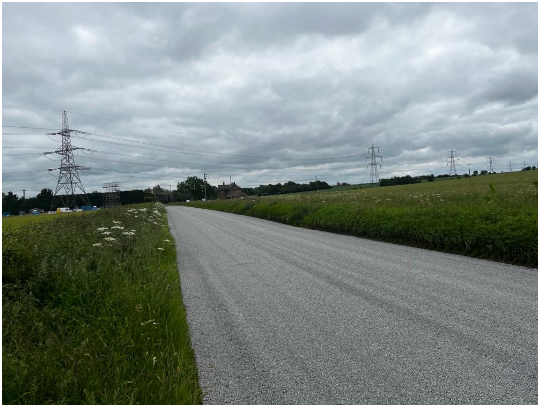
Completed Micro Surfacing – High Street, Landbeach – 2023/24
