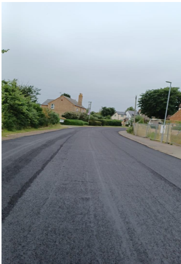
Completed Micro Surfacing – High Street, Landbeach – 2023/24
