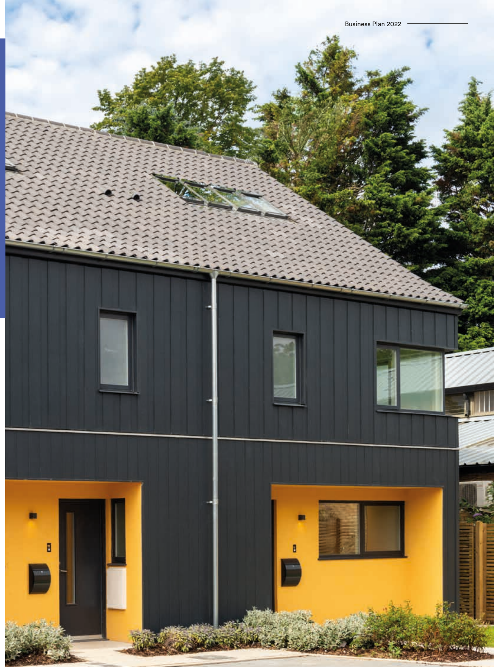
Completed house at our site at Ditton Walk
