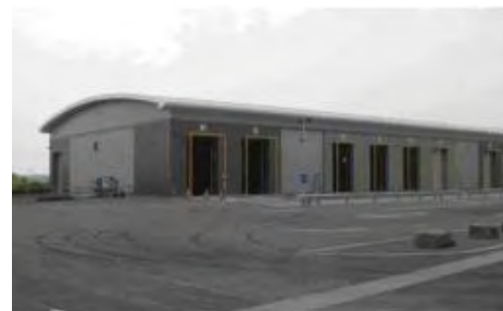
Built form of Alconbury Waste Transfer Station
