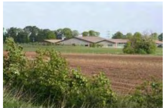
A good example of a large scale building in a rural setting
