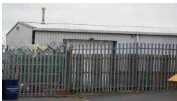
An example of unsuitable boundary treatment
