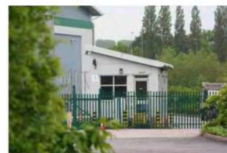
A simple gatehouse, but let down by the utilitarian security gates
