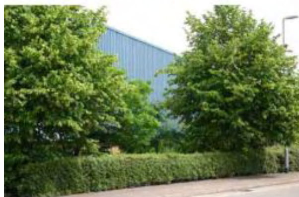
Landscape treatment can soften a simple building facade
