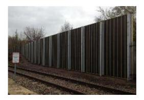
Figure 2: Example of an acoustic fence alongside a railway line
