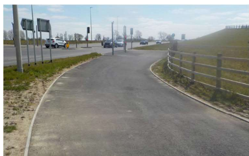
Figure 10 – View looking at controlled crossing
