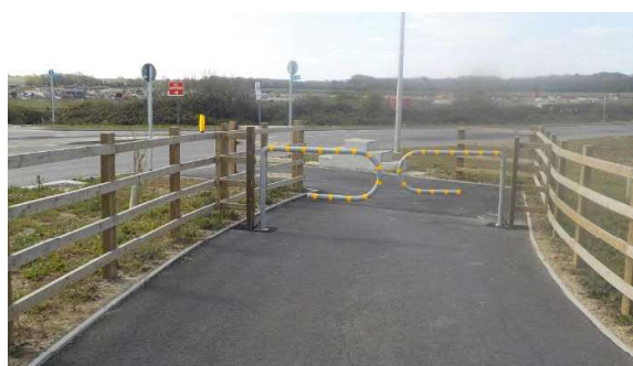
Figure 7- View looking towards uncontrolled crossing
