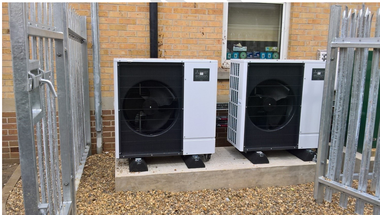
Figure 9. Air source heat pumps at Cottenham Library
