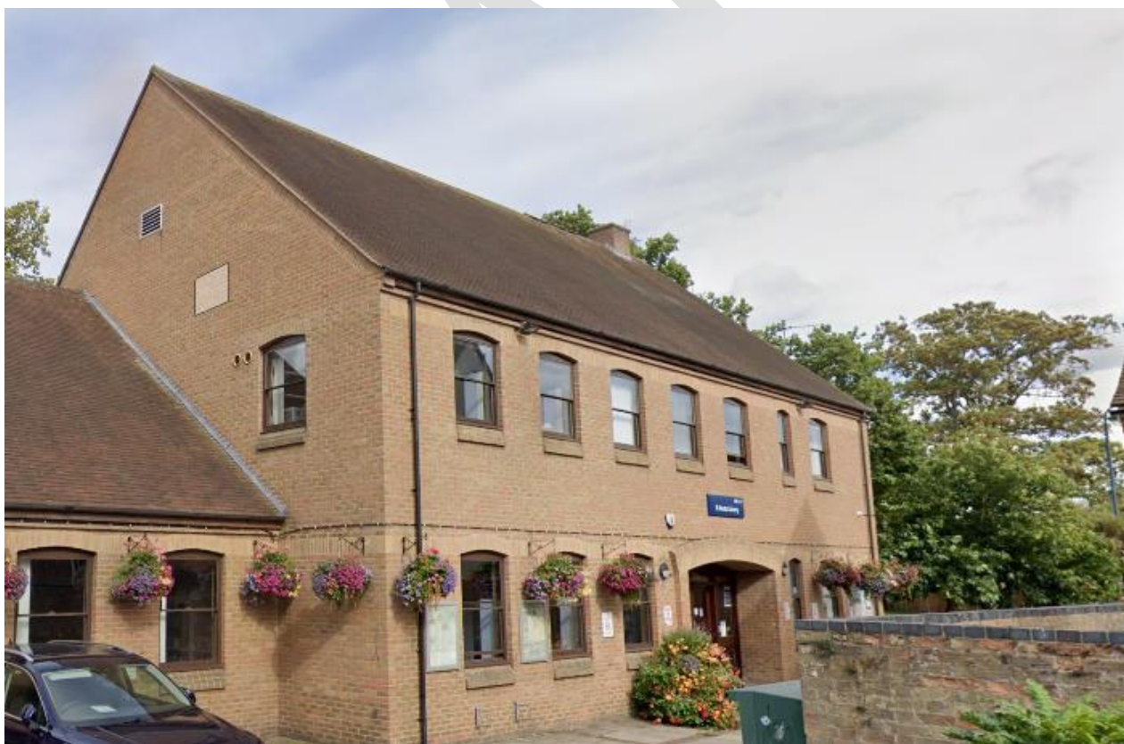
Figure 11. St Neots Library, which is now heated by air source heat pumps
