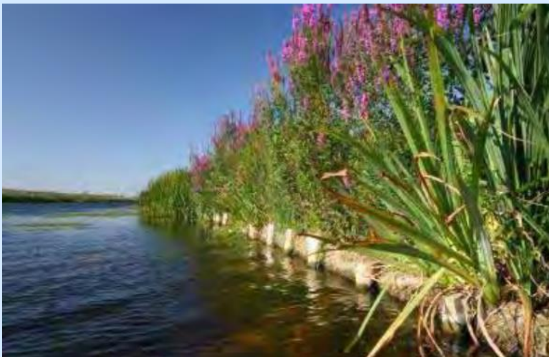
Coir rolls at Sixteen Foot River Credit: Cliff Carson
