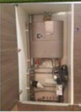
The HIU fits into a kitchen cupboard. It may replace an existing boiler and water heater, or these may be retained in addition to the HIU.
