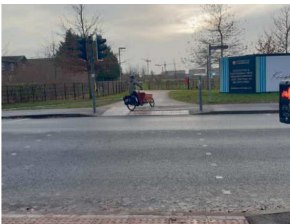
Photo 2: Toucan crossing for cyclists and pedestrians between Darwin Green and Eddington developments.
