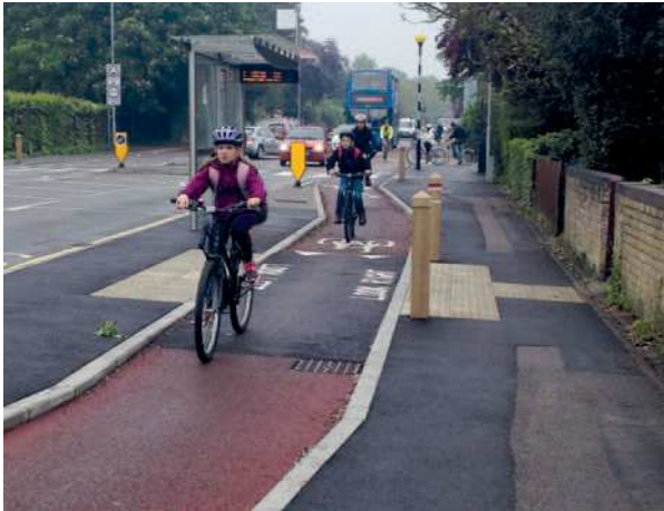
Photo 36: Cycle by-pass at bus stop, Huntingdon Road, Cambridge.
