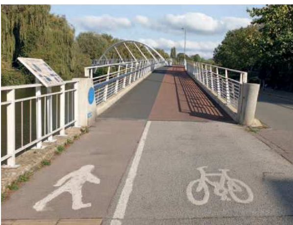
Photo 7: Riverside bridge linking a new development in Chesterton, Cambridge, to the existing cycle network to facilitate journeys to the city centre and station.
