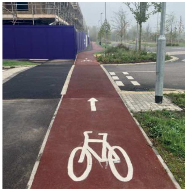
Photo 17: Side road treatment, Waterbeach.
