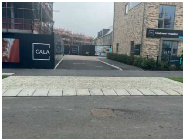
Photo 12: Continuous footway across a side road in Waterbeach.
