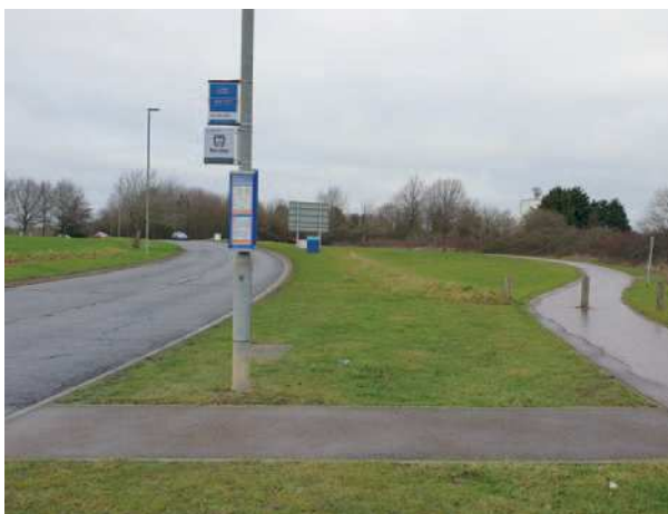
Photo 39: Section of footway across verge to access bus provided retrospectively several years after bus stop became operational, Cambourne.
