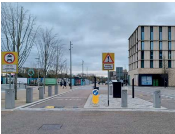
Photo 24a: Use of rising bollards to act as a modal filter allowing only buses, taxis, emergency vehicles and cyclists, to use the main high street through the development Monday – Friday, 7am – 7pm, Eddington, Cambridge.
