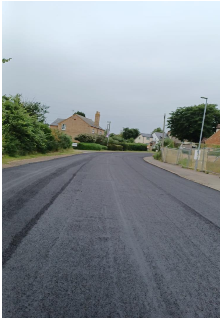
Completed Micro Surfacing – High Street, Landbeach – 2023/24
