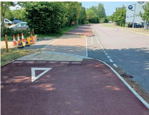
Photo 21: Priority given to vehicles accessing car park rather than those using the shared path, (note: in this urban location cyclists and pedestrians should also be segregated) Cambourne, South Cambridgeshire.
