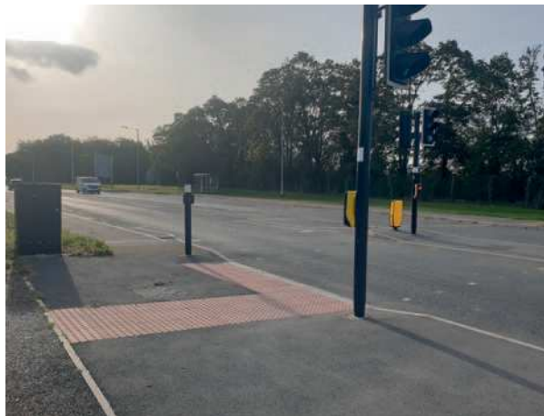
Photo 9: Connection to the existing shared path and bus stop from Babraham Research Park, Cambridge.
