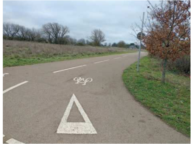
Photos 23a & 23b: Junction of off-road shared paths where segregation and give way lines have been introduced retrospectively to reduce conflict between users in Eddington, Cambridge.
