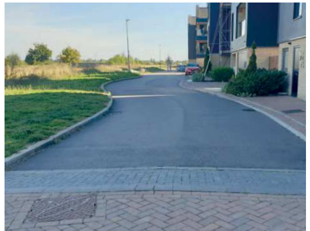
Photo 27b: The same road where the design could better reflect the shared space concept as this layout looks to users as if the footway is blocked by planting, Clay Farm, Cambridge.
