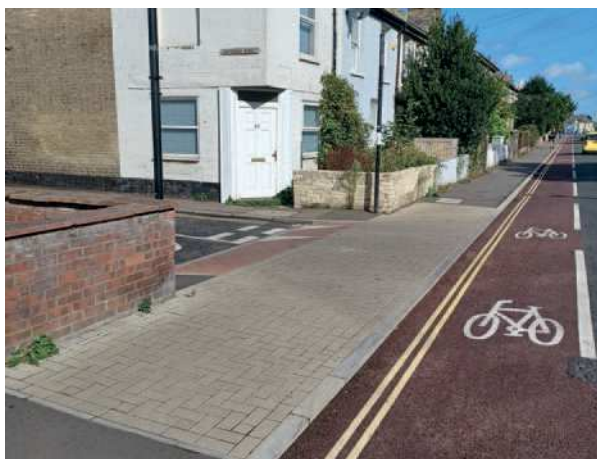
Photo 13: Continuous footway for pedestrians, Histon.
