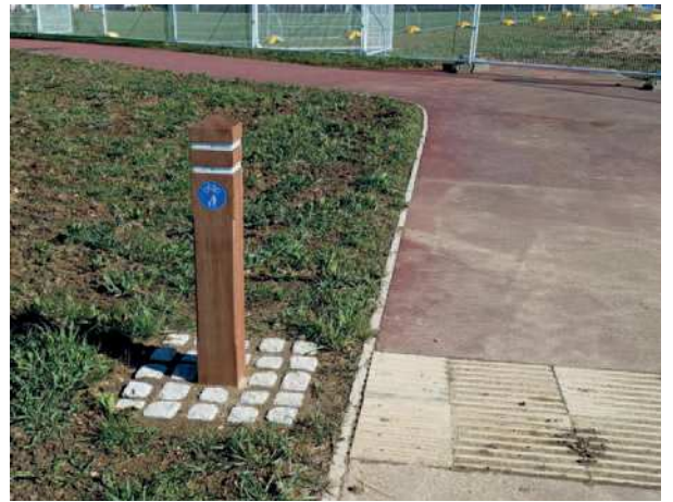
Photo 49: Less obtrusive shared use signage on wooden bollard rather than larger post, West Cambourne.
